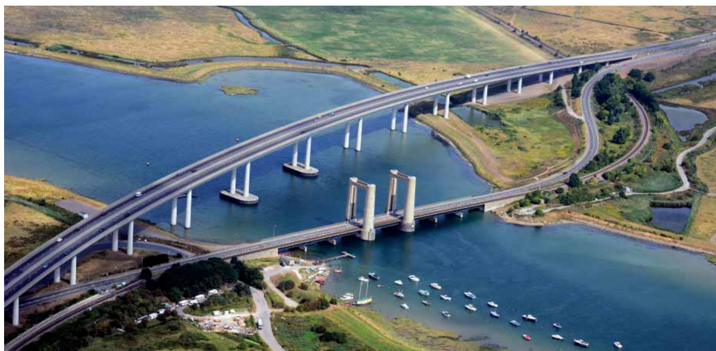
Image of the new Sheppey Crossing, with the Kings Ferry Transporter Bridge in the foreground: two pieces of key 20th and 21st century transport infrastructure linking the island and mainland parts of Swale Borough.
