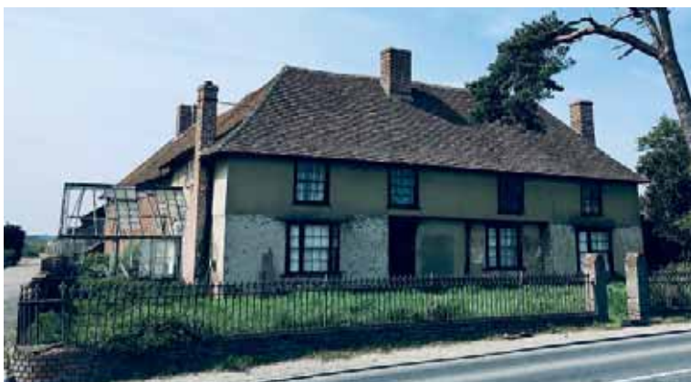
Radfield House, Teynham – at risk grade II listed building, disused and neglected by its large business owner.
