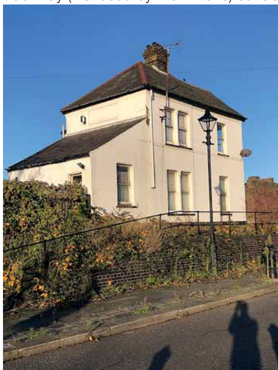
Pier Toll House, Sheerness (a non-designated heritage asset)
